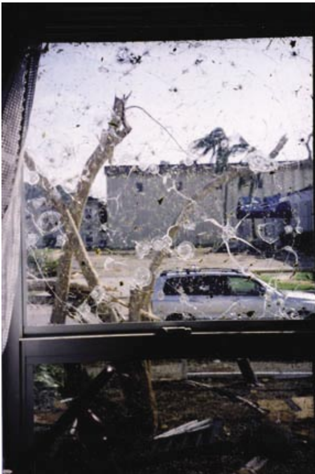
This image shows the shattered but intact window in the front of Liz Hutchinson's home.
